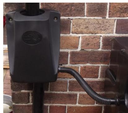
4) Now your diverter is installed it's time to connect it to your tank. To do this, simply screw in/insert the diverter hose end into the pre-fitted brass eyelet at the top of your tank (available at either end). You will need to pierce the required eyelet with a drill bit, please take precautions when doing this.
